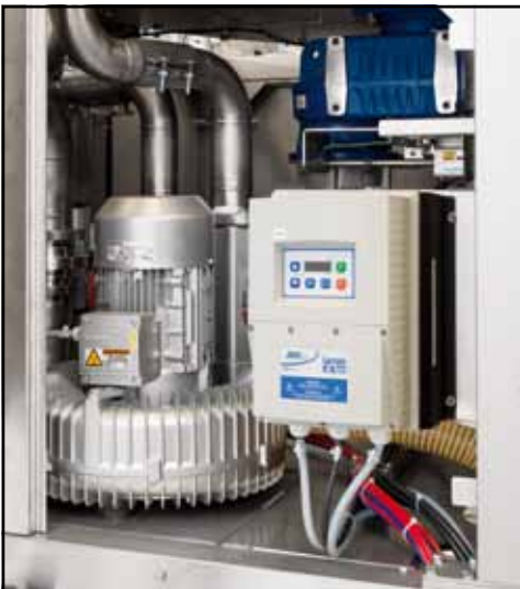
On-board vacuum pump and inverter
